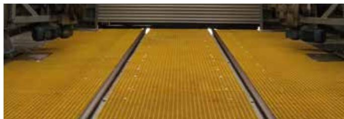
Track Pan installed at Perth Station as part of a carriage washing facility.
